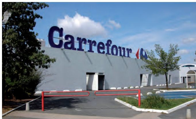
Carrefour's exit from Russia – after only two store openings – seems premature
